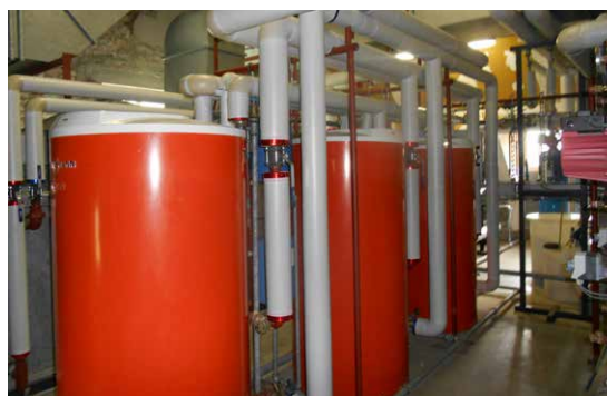
The biogas unit in Ochain is connected to larger environmental initiatives.
